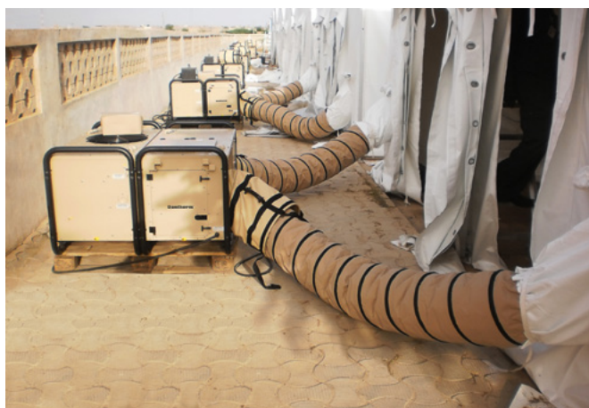
Installation with the air ducts
