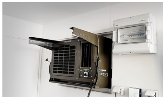
Container installation - inside view
