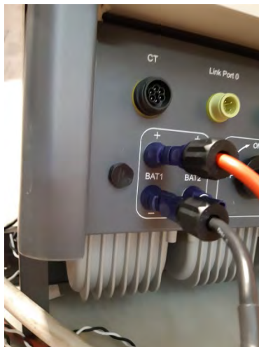
Figure 48 - Inverter-side DC power connection with a single battery input populated
