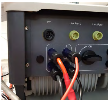
Figure 87 - Inverter-side DC power connection with two battery inputs populated
