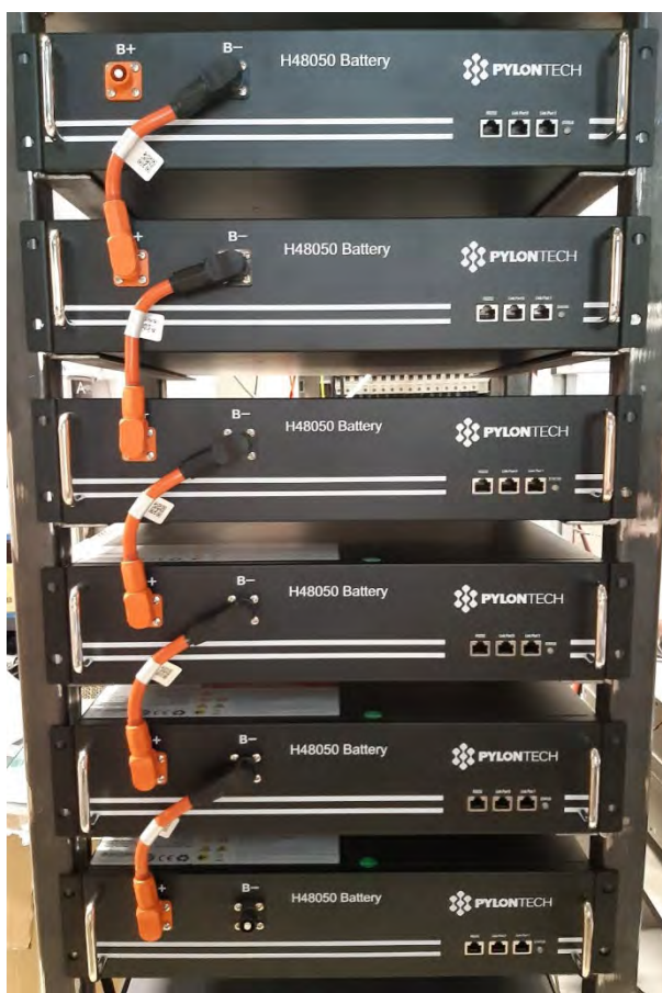
Figure 42 - Power cable between battery modules
