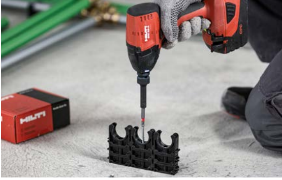
1 The REHAU pipe clip spacers.
