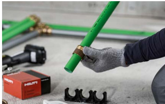
10 Slide on the compression sleeve. The chamfered end needs to face the fitting.
