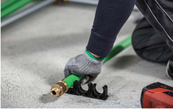
1 Pull the RAUPEX pipe out of the pipe clips.
