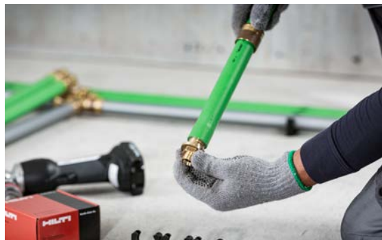
12 Push the fitting into the expanded pipe section.
