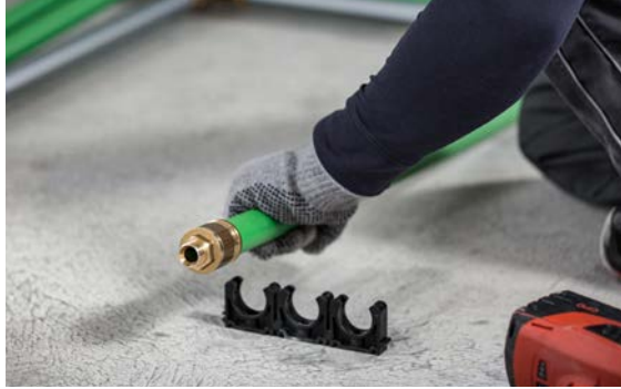
2 Remove the RAUPEX pipe.
