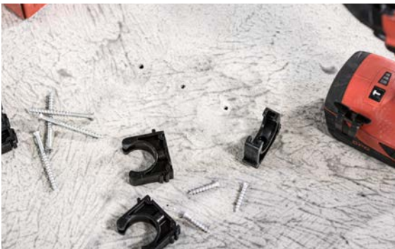
5 Then remove the REHAU pipe clips.
