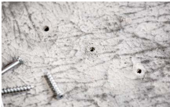
6 Small, drill holes remaining in the floor. They can be filled if required.
